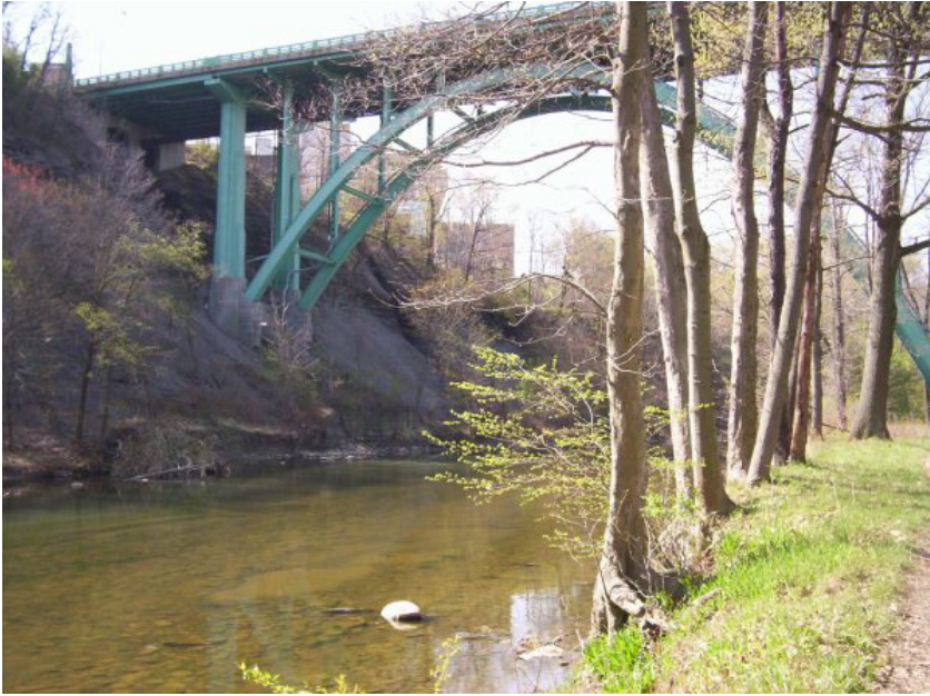
Figure 3: Bridge Near Fairview Park
